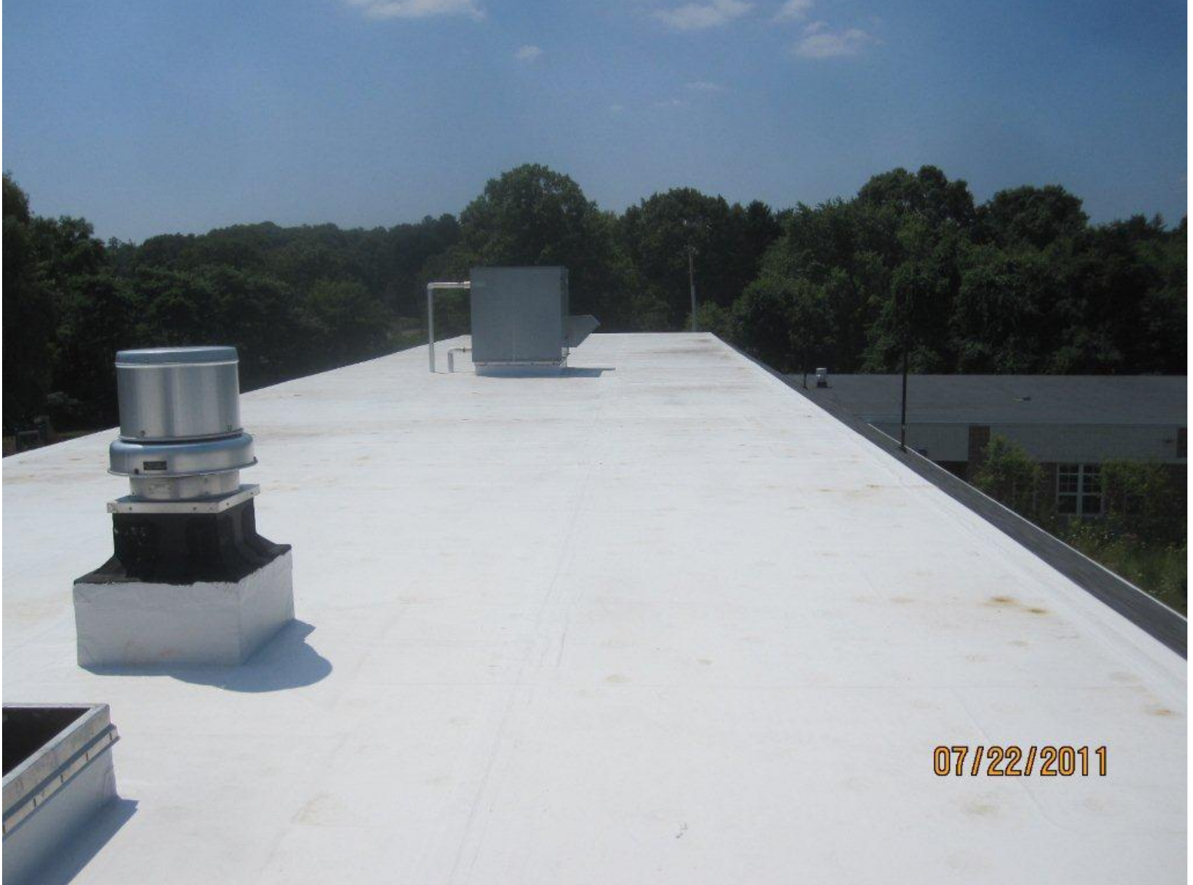
GLOVER ELEMENTARY SCHOOL ROOF COATING COMPLETED
