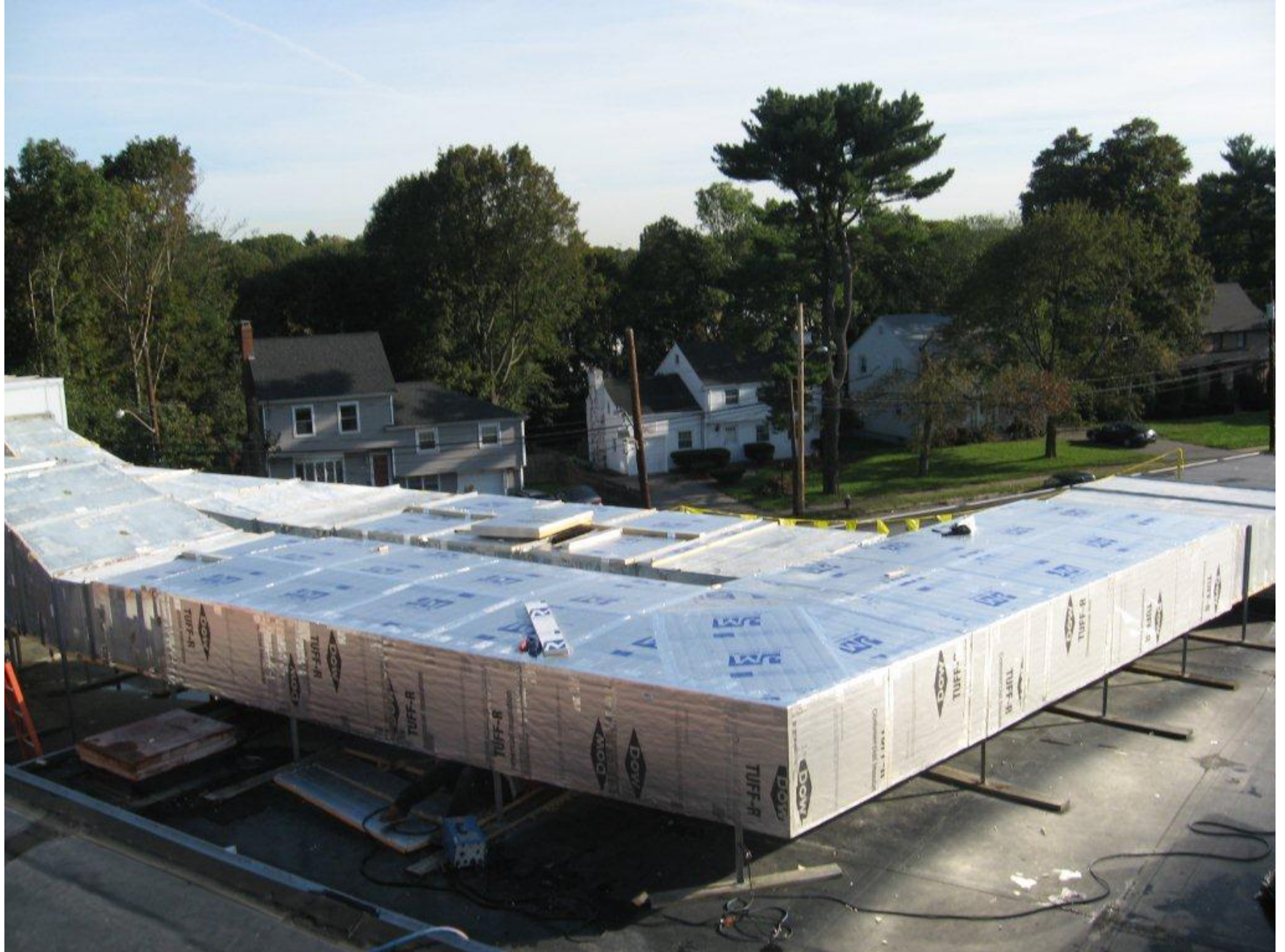
DUCT WORK UNDER REPAIR
